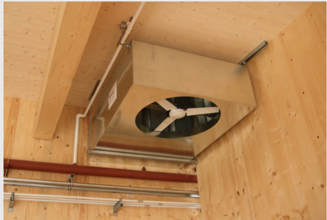
Example installation prior to construction of bulkhead
