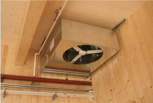
Example installation prior to construction of bulkhead
