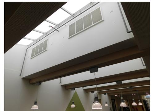
The Breathing Buildings e-stack A500 unit is an assisted atrium system. By providing a flow path through the building, it also aids the adoption of a natural ventilation strategy for the surrounding rooms. The innovative low-energy system can be deployed in
