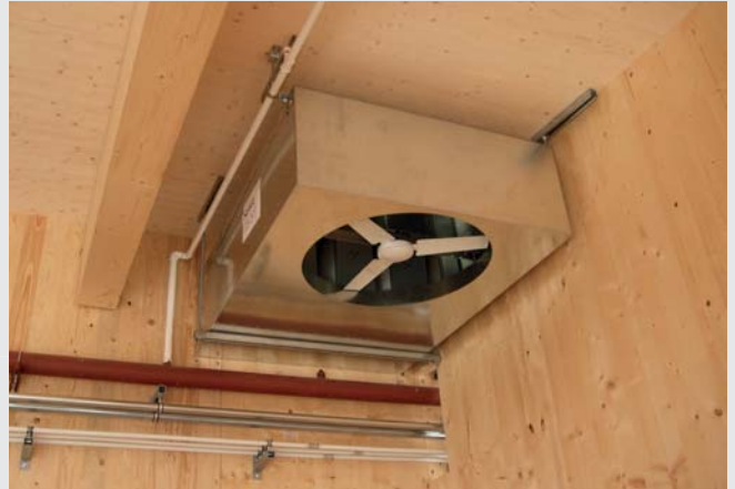
Example installation prior to construction of bulkhead
