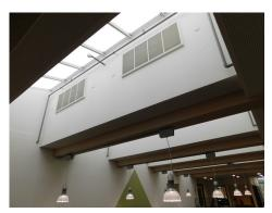
The Breathing Buildings e-stack A500 unit is an assisted atrium system. By providing a flow path through the building, it also aids the adoption of a natural ventilation strategy for the surrounding rooms. The innovative low-energy system can be deployed in
